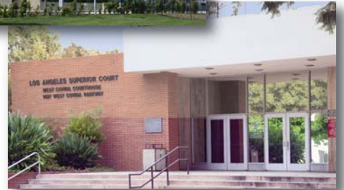
West Covina Courthouse
