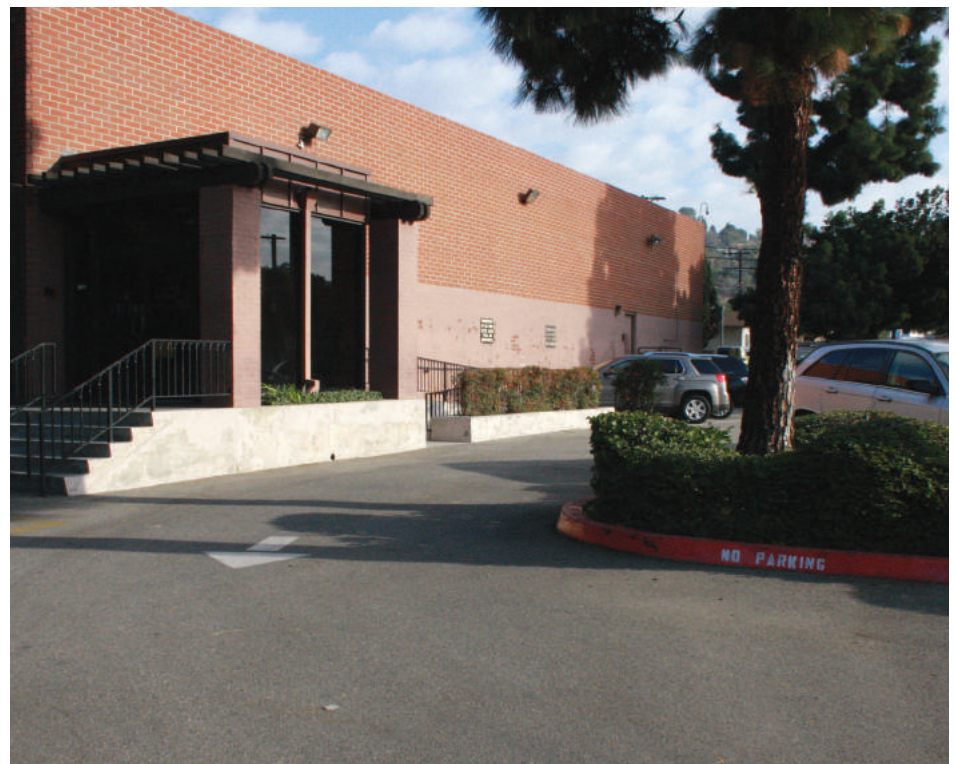
The Mental Health Courthouse before its closure in November 2016.
