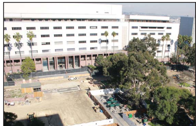
Civic Center Park under construction.
